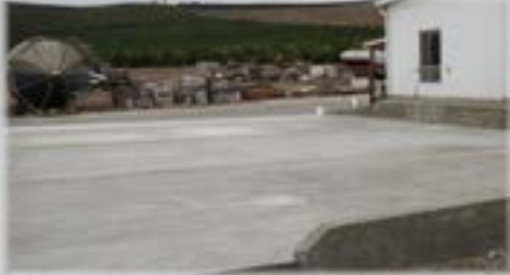
cement pad for new silos
